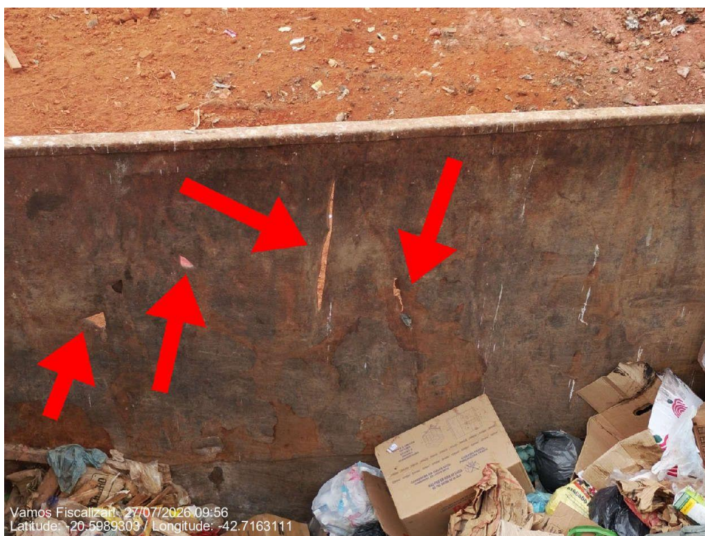
Rachaduras no container.
